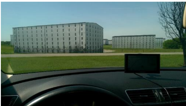
Rik Barns, Heavenly Hill Distillery
