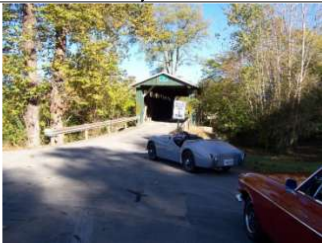
Parked at the Ballard Road Bridge – this bridge is original and still in decent shape, but does not support much traffic since the 4-lane US 35 cut Ballard Road. Temperature is up above 50 degrees by this time...
