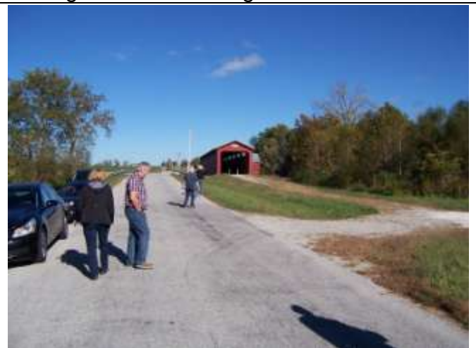
Engle Mill Road Bridge – a little walk from the place we parked on the road.
