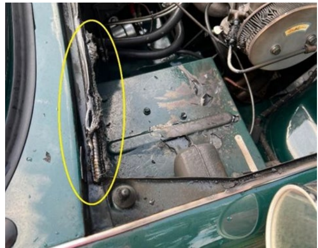
Melted seal strip that hindered hood opening
