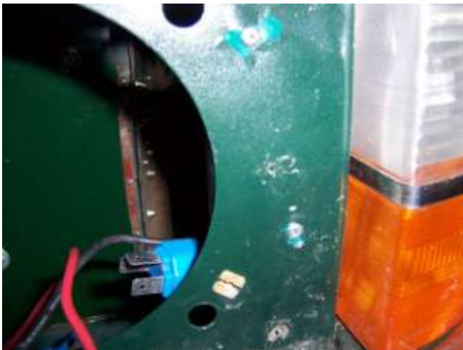
Driver's LED Power Converter Pop-riveted to back side of the front valence, driver's side. Evidently the paint here wasn't prepped good for that last respray....
