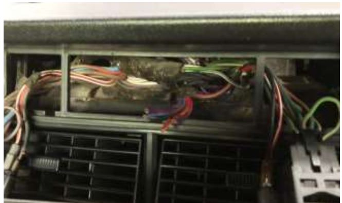
Issue 2: no fog light switch (cut off)
