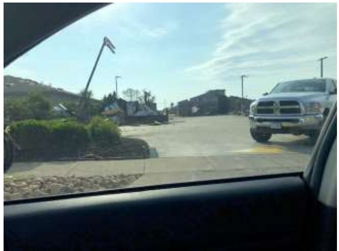
Mike Car Wash on North Fairfield was pretty much destroyed.
