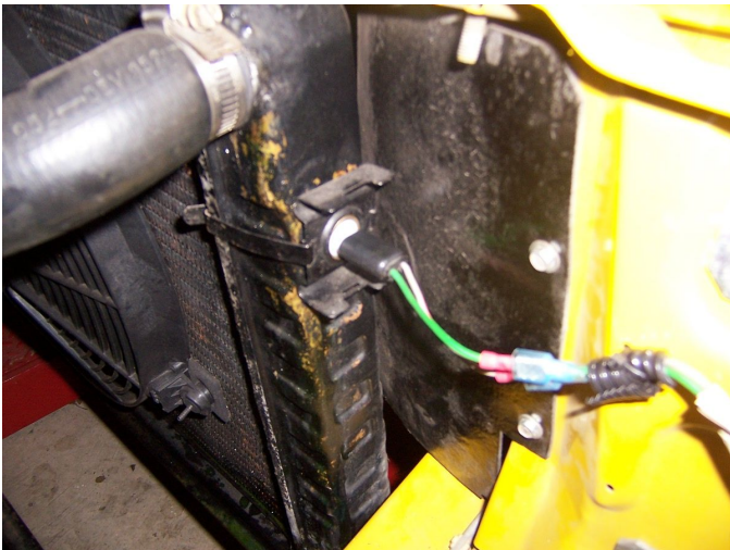
New-Old Fan Switch in place
