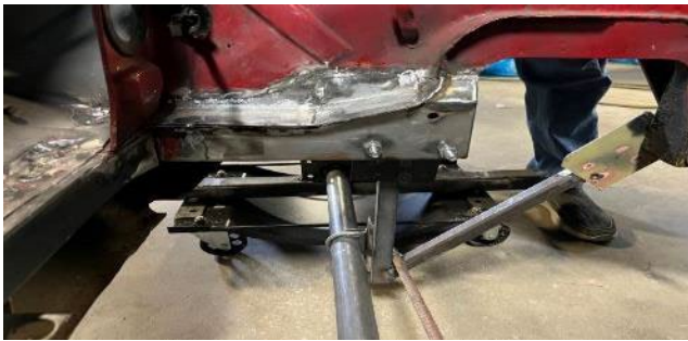
Picture of repair unpainted.
