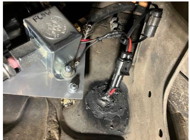
Black silicone sealant is your friend – instagrommet – the electrical connections at the pump.
