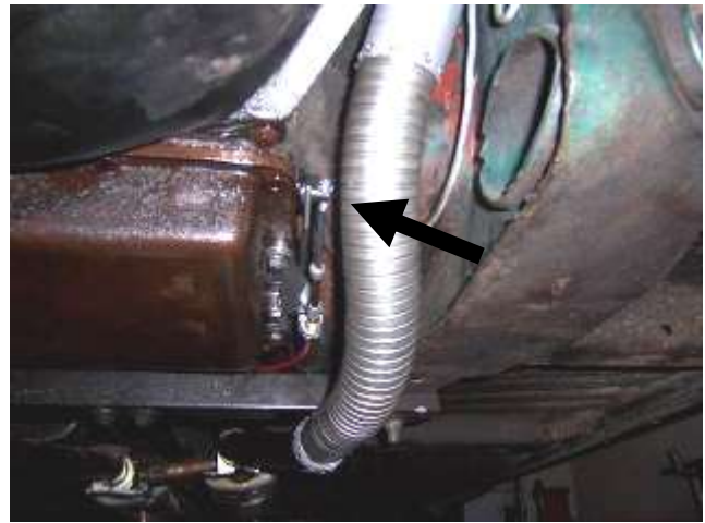
Flexpipe Installed – We Now Have Clearance Houston!
