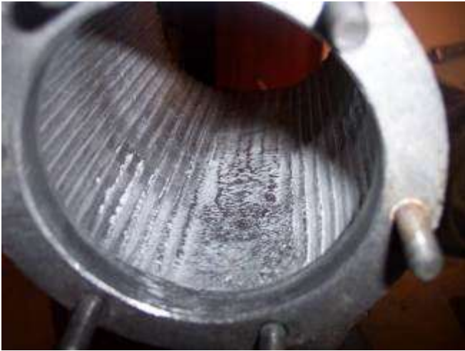
Removed enough metal at the bottom here to make the flat section round at the same circumference as the rest of the tunnel
