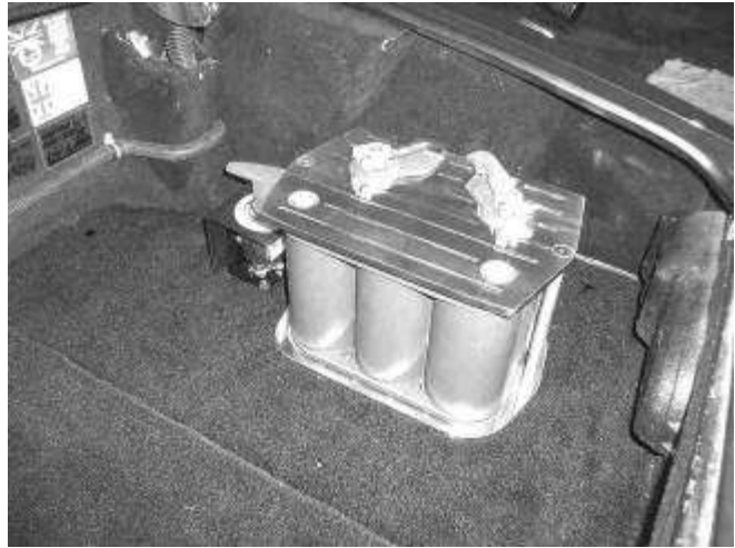
Optima Gel-Cell Battery and Cut-Off Switch Mounted In Trunk Close TO The Location Of The Battery That Was In The Car When I Got It, Without The Duct Tape!
