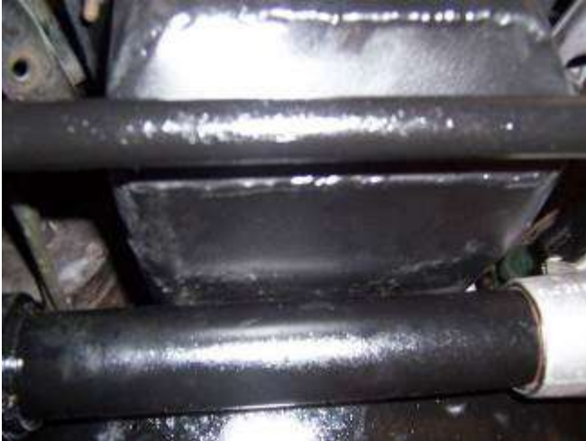
Close fit under the oil pan, almost too close!
