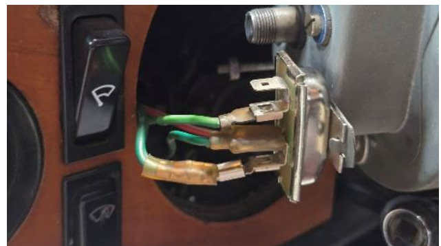
Getting this puppy out is a bit of a pain – the unit is attached to the back of the speedometer, and to get the speedo off is a royal pain due to no room for normal hands.
